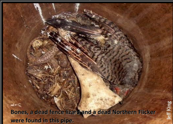
50 year old uncapped irrigation vent pipe.
